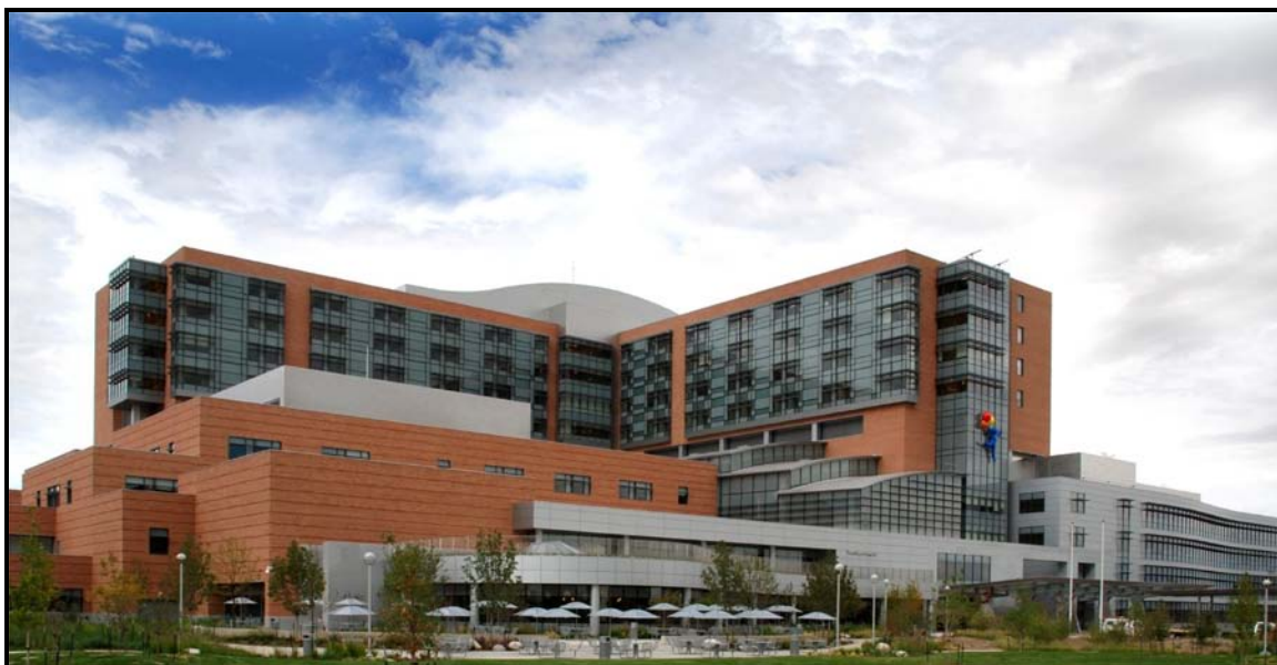
The Children's Hospital at Fitzsimons Medical Center, Aurora, Colorado (Source: The Children's Hospital Foundation)
