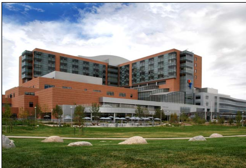
Children's Hospital Colorado at Anschutz Medical Campus Aurora, Colorado (Source: Children's Hospital Colorado)
